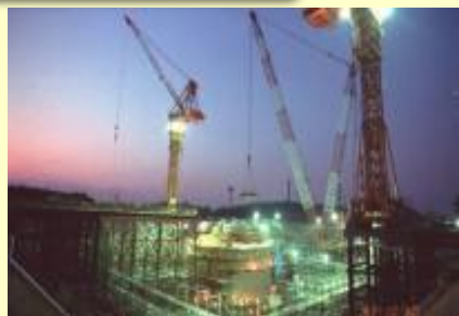
Installation of Reactor Pressure Vessel
