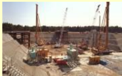
Start Construction Work
